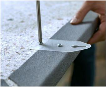
For the panel(s) that will be used for the top row, install the hang tabs just below the top edge. Install the hang tabs with equal distances from the top edge of the panel(s).
